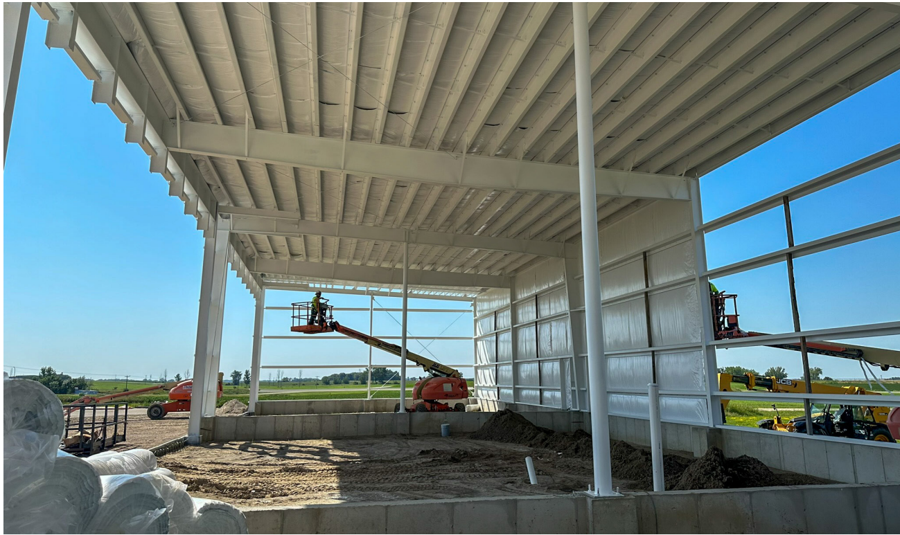
TKDA developed a four-unit premanufactured steel hangar structure that is flexible in the size and number of aircraft that can be accommodated
