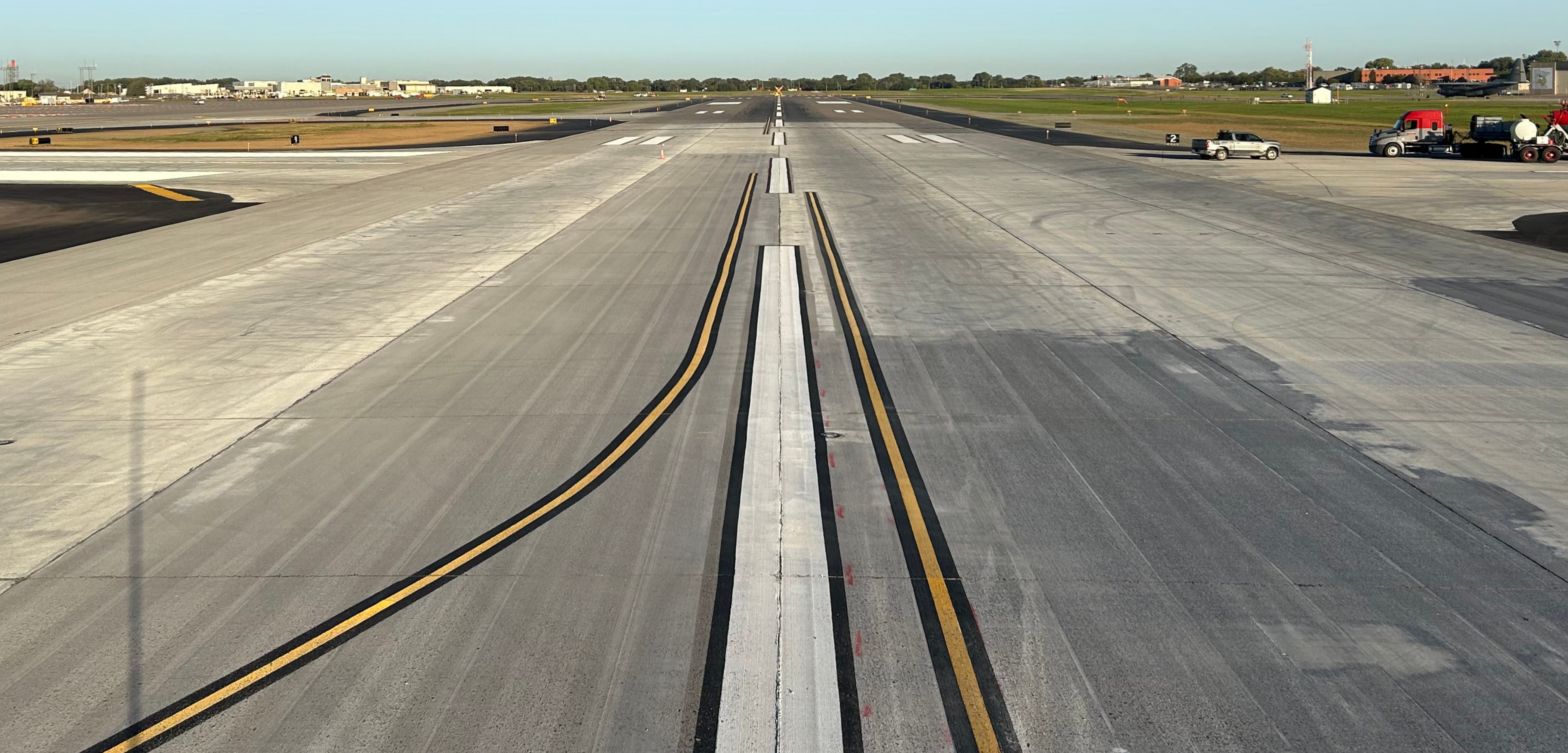
TKDA regraded the safety area adjacent to Runway 12L-30R along both sides of the entire length of the runway, requiring close coordination with the taxiway and intersection work
