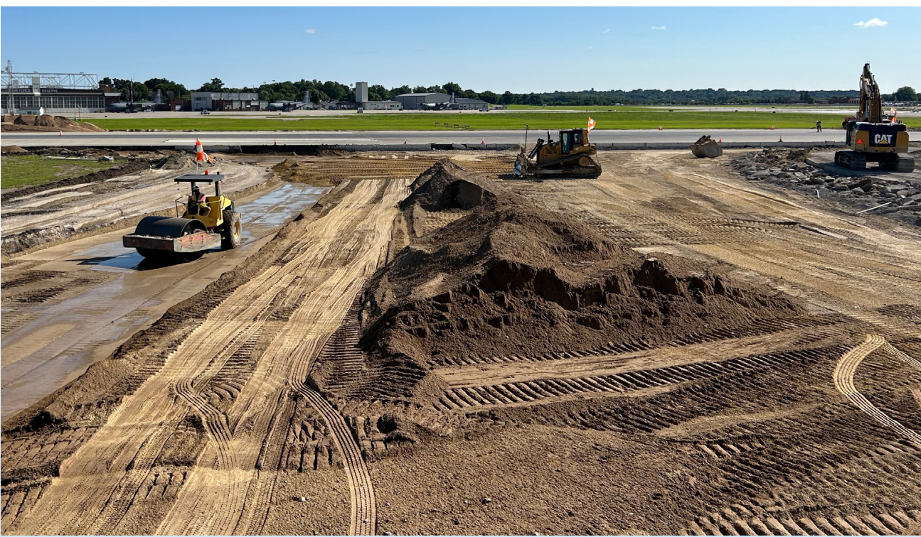
TKDA regraded the safety area adjacent to Runway 12L-30R along both sides of the entire length of the runway, requiring close coordination with the taxiway and intersection work
