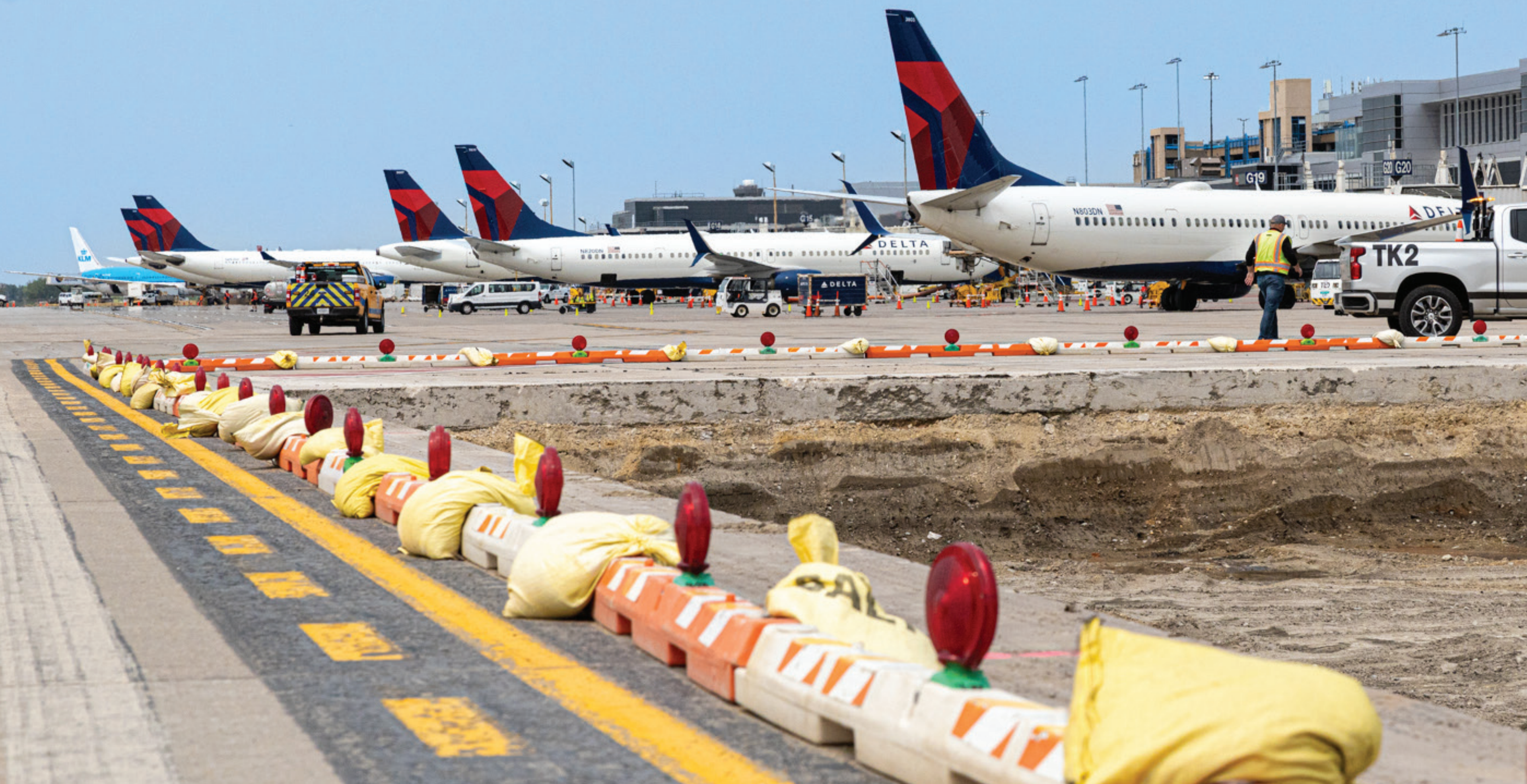
A dedicated glycol sewer system was installed to capture aircraft deicing fluid and separate it from the stormwater system, where it could cause harmful effects to aquatic species
