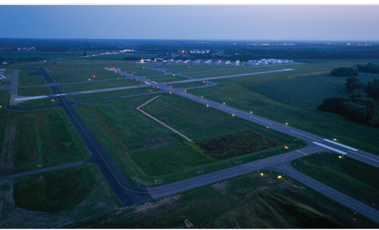
The project included all new LED edge lighting and signage.
