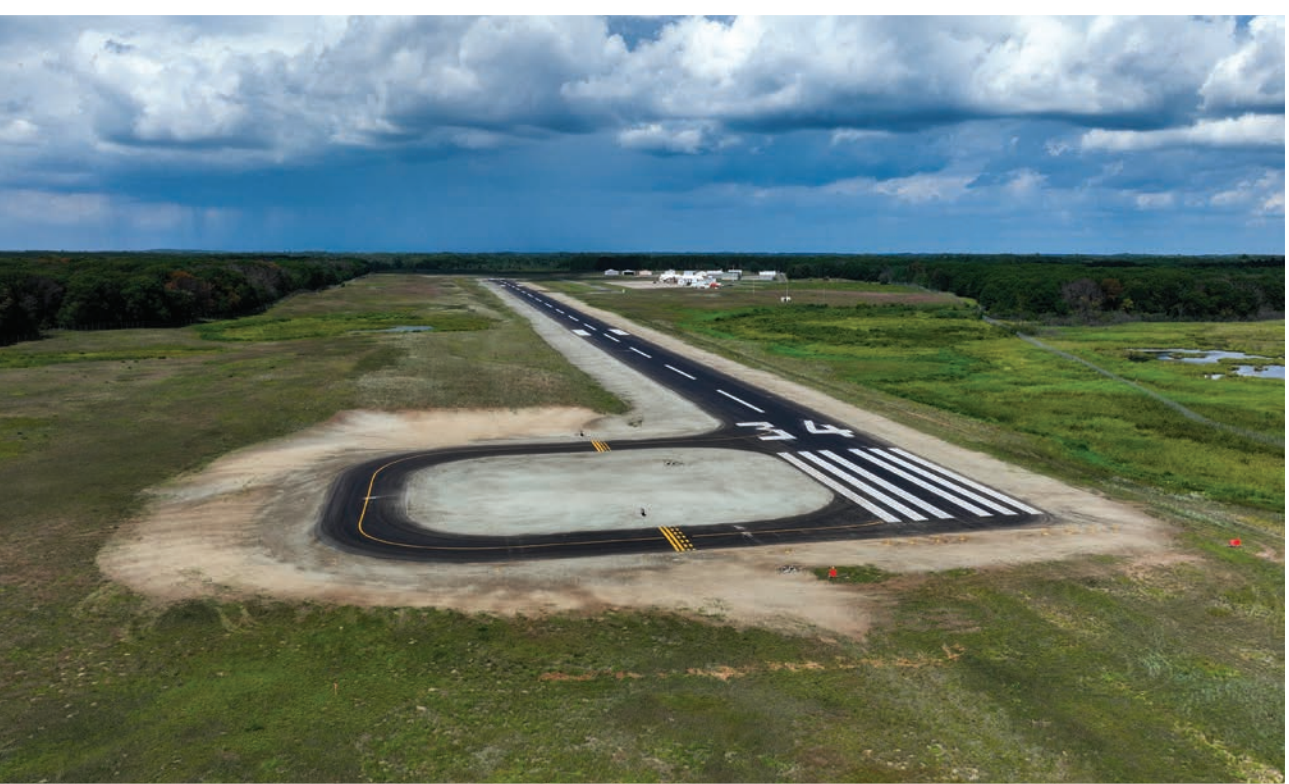
The project included the addition of a taxiway turnaround to the Runway 34 end, enhancing traffic flow and safety.
