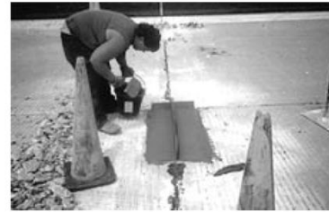
Figure 12.1. A partial-depth repair spanning both sides of the joint.
