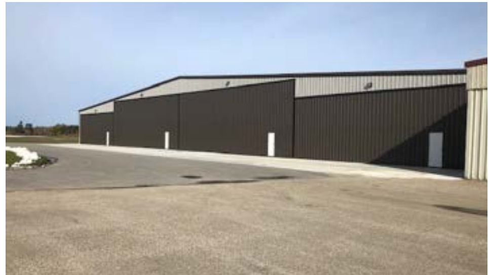
Multi-Bay Hangar with Different Door Heights
