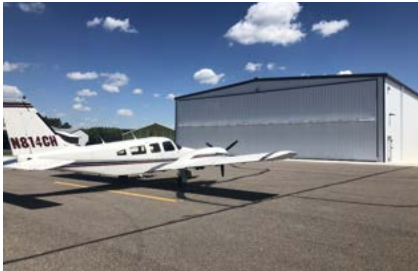
Multi-Plane Box Storage Hangar
