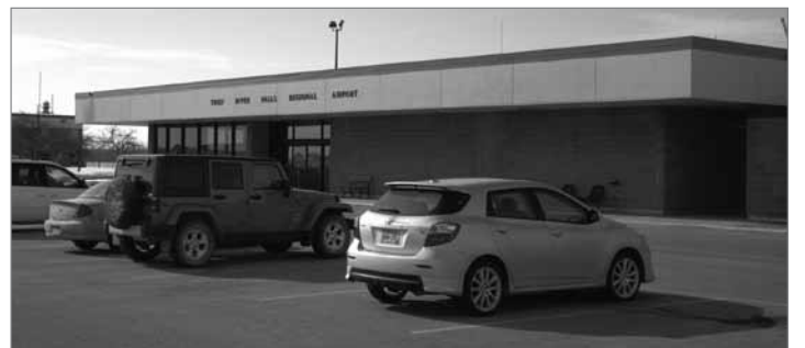
The Thief River Falls Airport terminal
