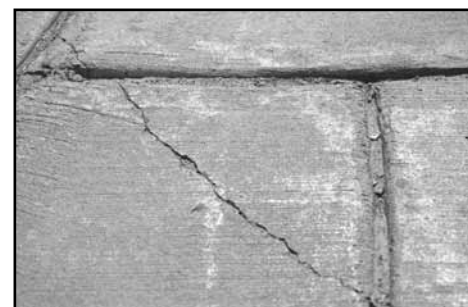
Corner crack
