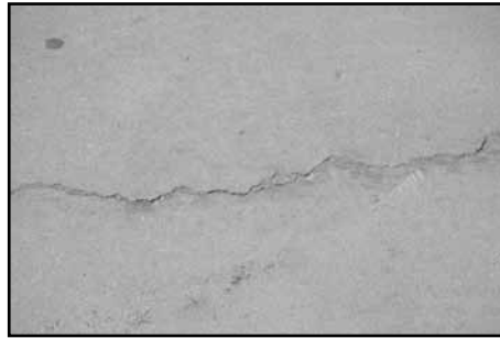
Mid-panel crack
