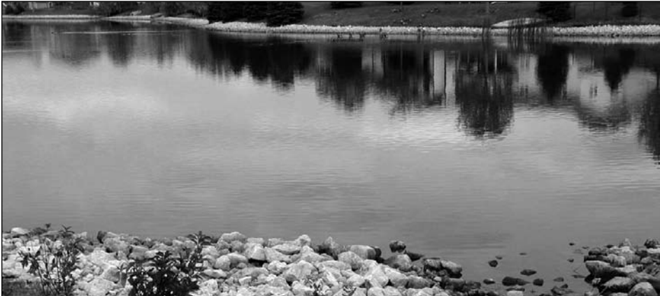
Fig. 1. Detention ponds temporarily store and treat storm water until it can be discharged.
